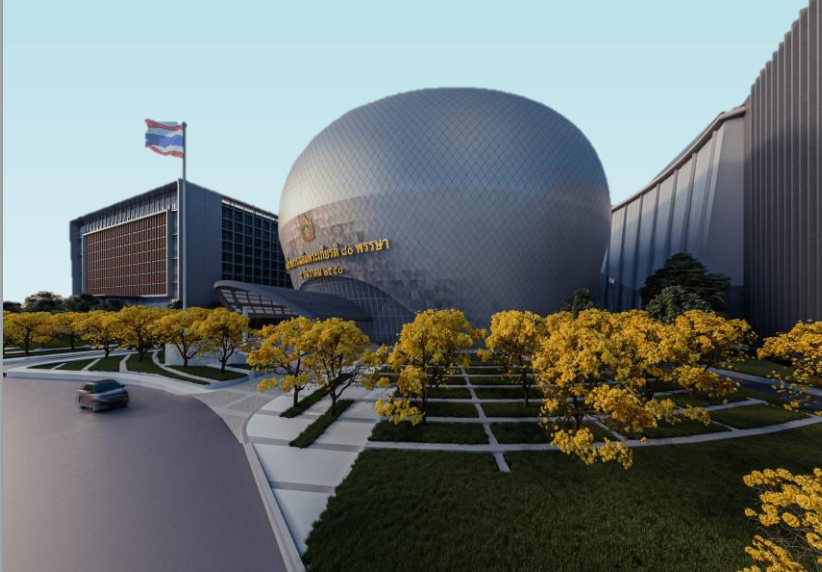
Government Center Zone C, DCS Project
