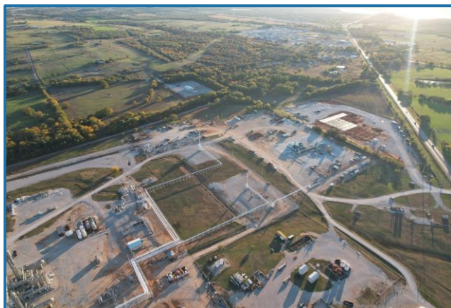
A pipeline seamlessly transports CO 2 from EnLink Midstream's processing plant to the BKV compressor facility for underground sequestration.
