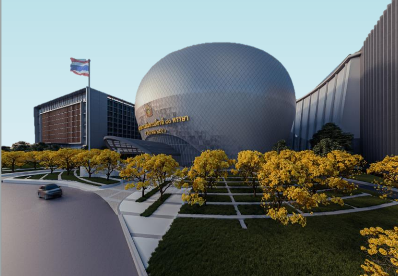
Government Center Zone C, DCS Project
