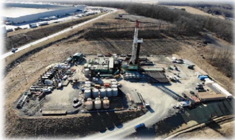
Drilling Operations – P&G Warehouse Pad
