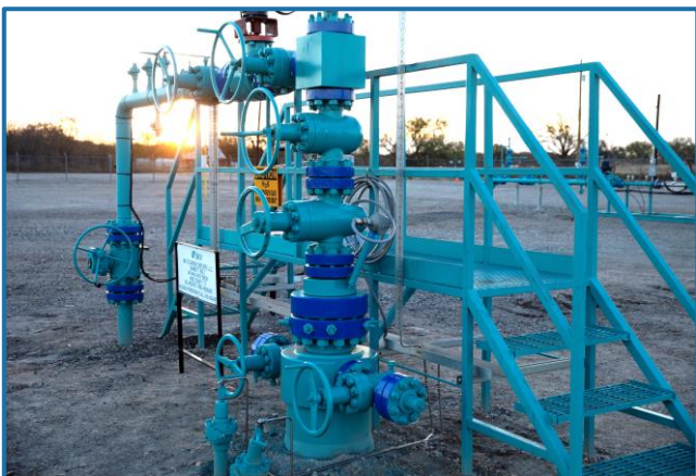
The well head at the BKV Barnett Zero underground injection control well.
