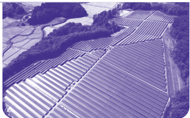
Yabuki Solar Power Plant in Fukushima Prefecture, Japan
