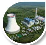
Coal-fired power – IPPs
