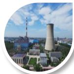
Combined Heat & Power
